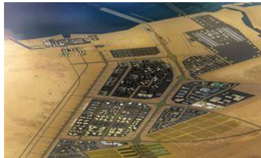
Top – An artists impression of Sowwah Island (Central Business & Financial District) Below – KIZAD (Khalifa Industrial Zone Abu Dhabi) masterplan
